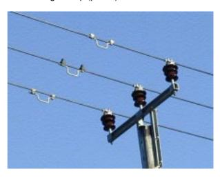
Picture 4. suspension pole with earthing stirrups.
